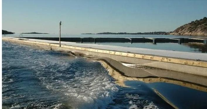
*Fig. 2. A concrete pier reinforced with basalt fiber from the Swedish company SF Pontona*
