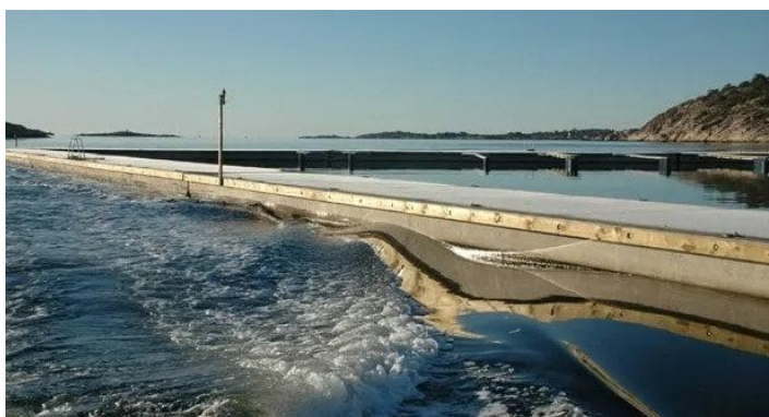
Fig. 2. A concrete pier reinforced with basalt fiber from the Swedish company SF Pontona
